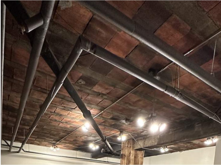
Exposed clay tile ceiling from the one-way clay tile joist system.
