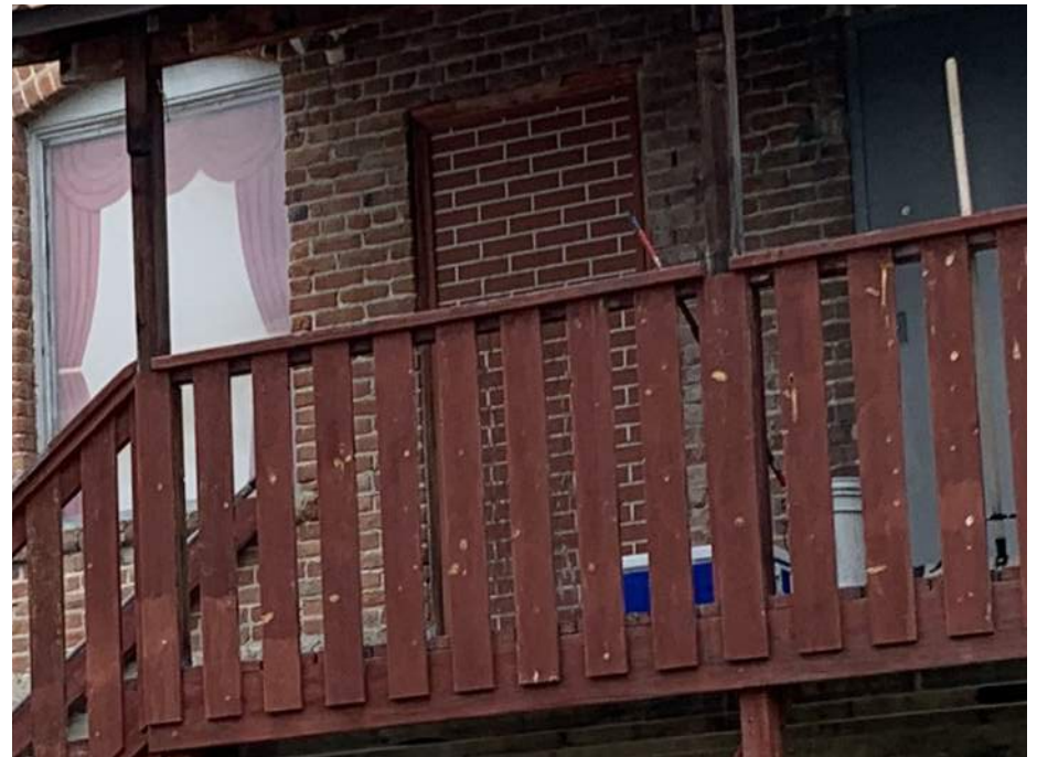
Previous door opening infilled with masonry at the exterior west egress stair.
