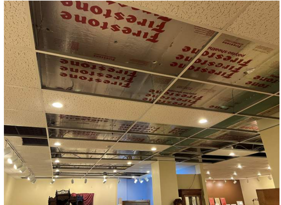
First floor ACT ceiling & insulation.
