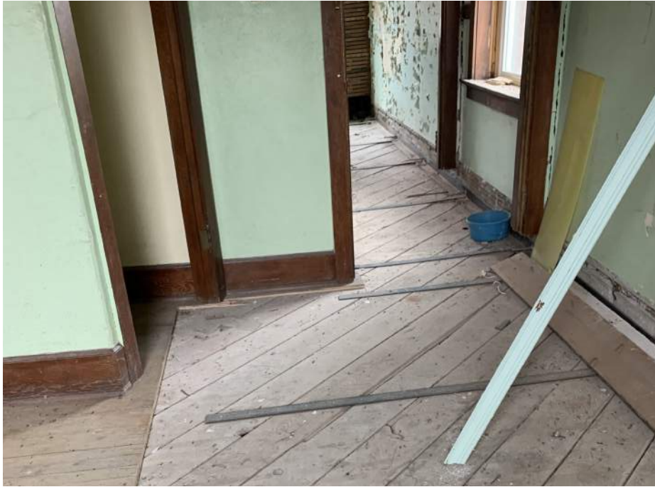
Third floor structural strapping.
